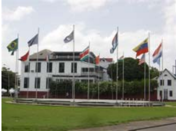
Paramaribo, Historic center
